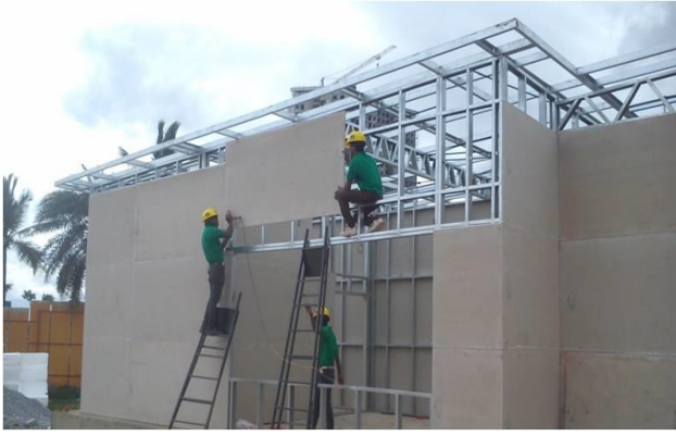
Figure 8: LGSFS on-site assembly
