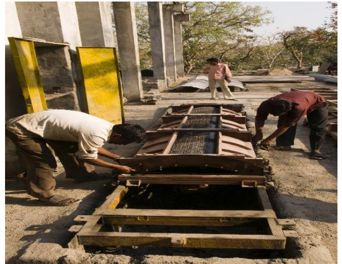
Figure 7: Ferro-cement roofing channels (on-site production)
