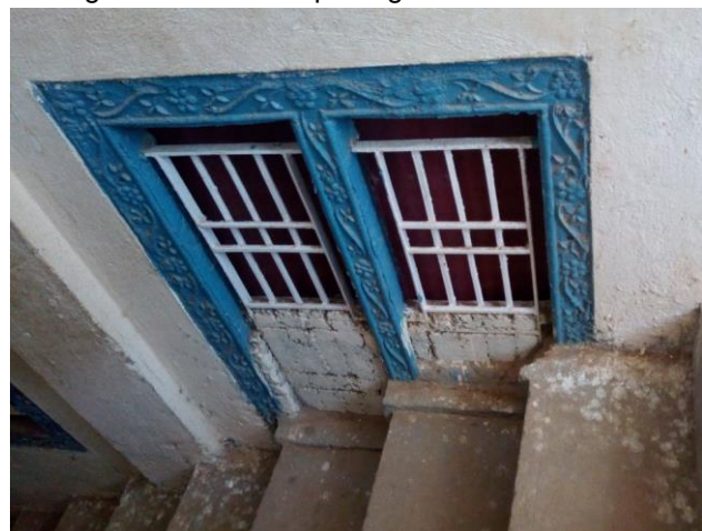
Figure 2: Window opening onto the staircase
