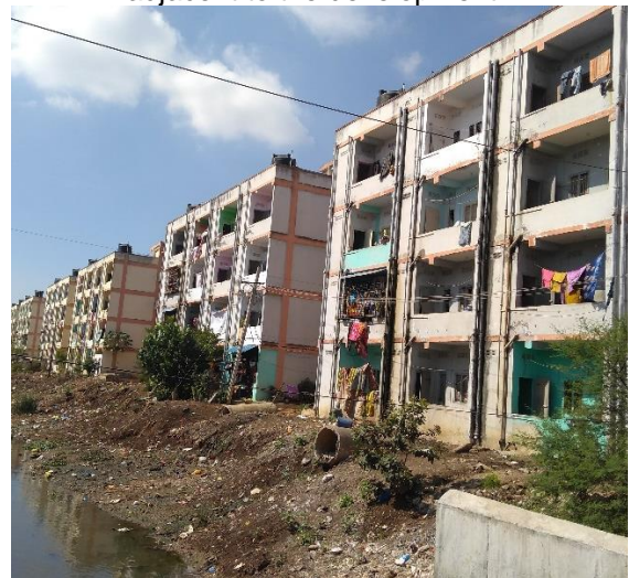
Figure 4: Sewage water accumulated on plot adjacent to the development
