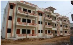
EWS housing in Jaipur, Rajasthan - RCC frame, brick
