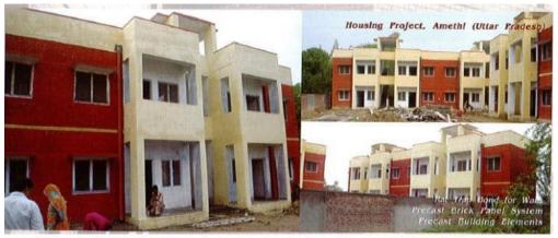
LIG housing in Uttar Pradesh - using Rat-trap bond walls and Precasat brick panel system
