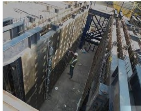
Figure 02: Battery Mould
